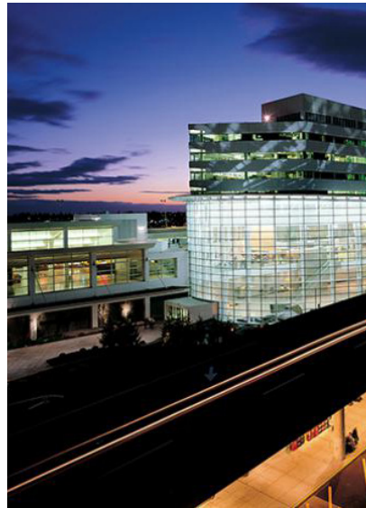
SEA-TAC INTERNATIONAL AIRPORT
